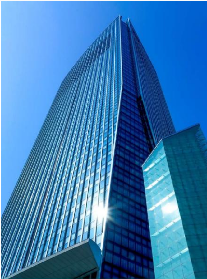
Toranomom Hills Mori Tower
