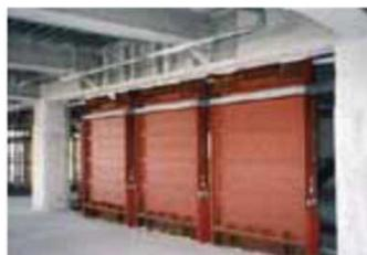
Viscous seismic damping wall
