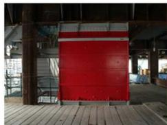
Viscous seismic damping wall
