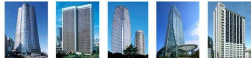
Roppongi Hills Mori Tower ARK Mori Building Atago Green Hills (MORI Tower) Toranomon Hills Mori Tower Holland Hills Mori Tower
