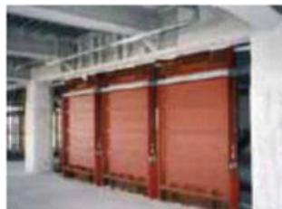
Viscous seismic damping wall
