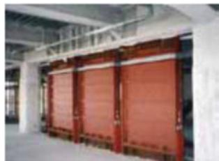
Viscous seismic damping wall
