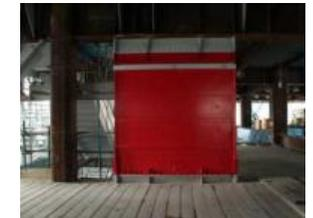
Viscous seismic damping wall
