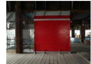
Viscous seismic damping wall
