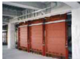
Viscous seismic damping wall
