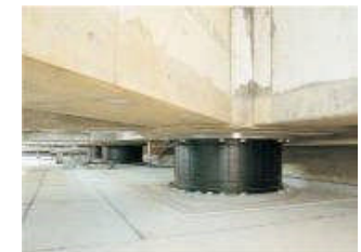
Seismic isolators
