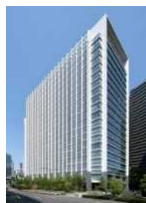
ARK Hills South Tower
