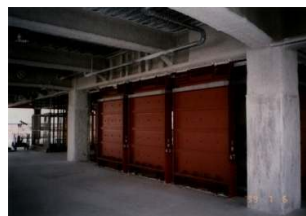
Viscous seismic damping wall
