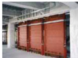
Viscous seismic damping wall
