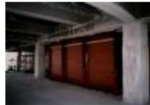
Viscous seismic damping wall
