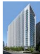
ARK Hills South Tower
