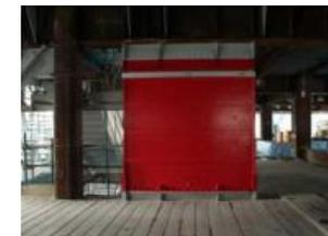
Viscous seismic damping wall
