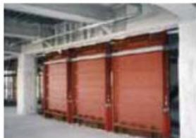
Viscous seismic damping wall
