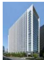
ARK Hills South Tower
