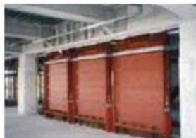
Viscous seismic damping wall
