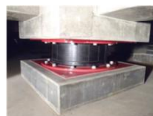
Seismic isolators
