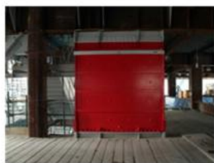
Viscous seismic damping wall
