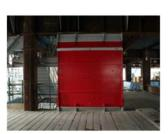
Viscous seismic damping wall
