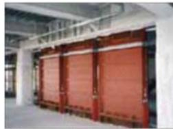
Viscous seismic damping wall
