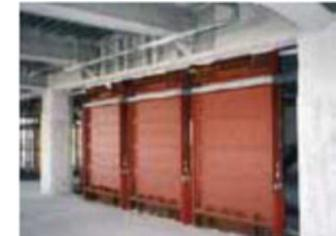
Viscous seismic damping wall
