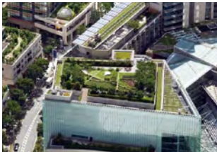
Rooftop garden(Roppongi Hills)
