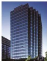
Koraku Mori Building
