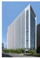
ARK Hills South Tower
