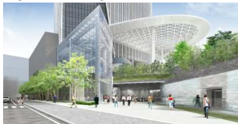
Main entrance (Note 2)
