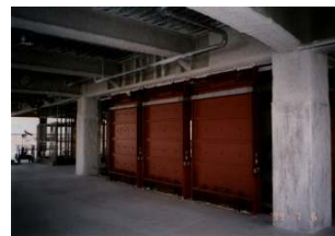
Viscous seismic damping wall
