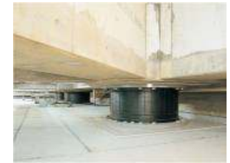
Seismic isolators
