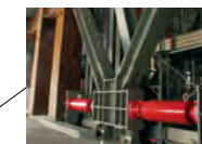
Oil dampers (516 units installed)
