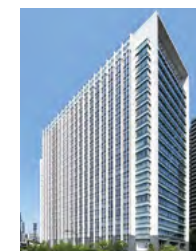
ARK Hills South Tower
