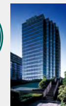
Koraku Mori Building
