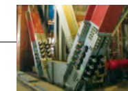
Brake dampers* (620 units installed)
