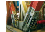
Brake dampers* (620 units installed)
