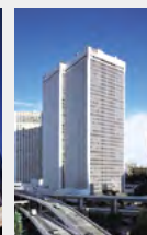
ARK Mori Building
