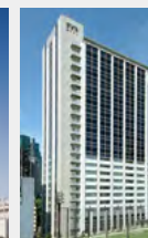
Holland Hills Mori Tower
