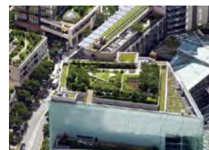
Rooftop garden(Roppongi Hills)
