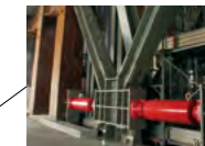
Oil dampers (516 units installed)
