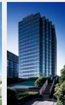
Koraku Mori Building
