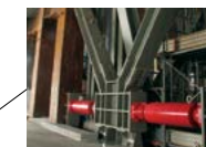
Oil dampers (516 units installed)
