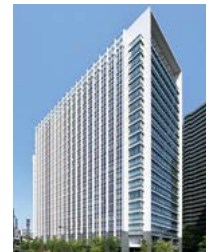
ARK Hills South Tower
