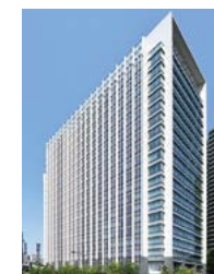
ARK Hills South Tower
