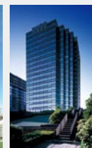
Koraku Mori Building
