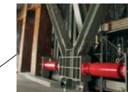
Oil dampers (516 units installed)
