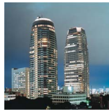
Atago Green Hills (completed: July 2001)
