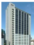
Holland Hills Mori Tower
