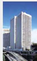
ARK Mori Building
