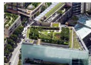
Rooftop garden(Roppongi Hills)
