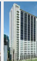
Holland Hills Mori Tower
