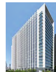
ARK Hills South Tower
