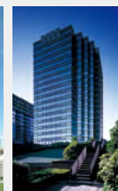
Koraku Mori Building
