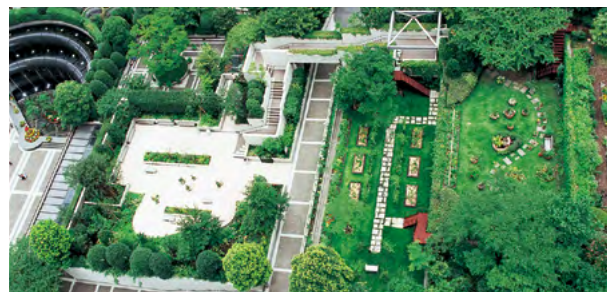
The roof top of Suntory Hall at ARK Hills
