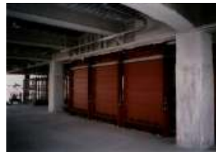
Viscous seismic damping wall
