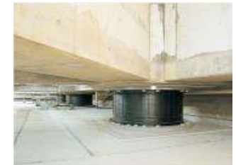
Seismic isolators
