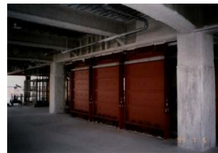
Viscous seismic damping wall
