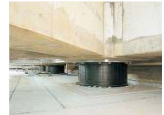
Seismic isolators
