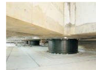
Seismic isolators
