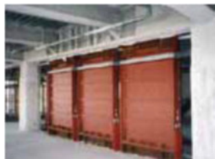
Viscous seismic damping wall
