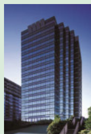
Koraku Mori Building
