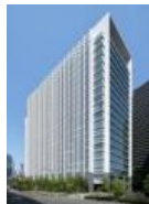
ARK Hills South Tower
