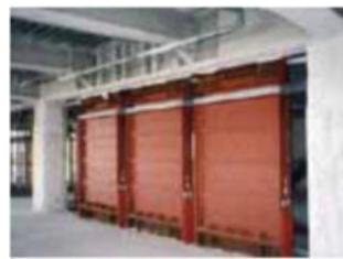
Viscous seismic damping wall
