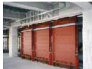
Viscous seismic damping wall
