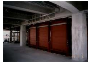
Viscous seismic damping wall
