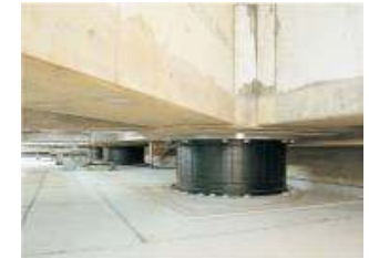
Seismic isolators
